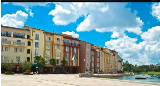
Colorful buildings house guest rooms at the resort and overlook the harbor.
